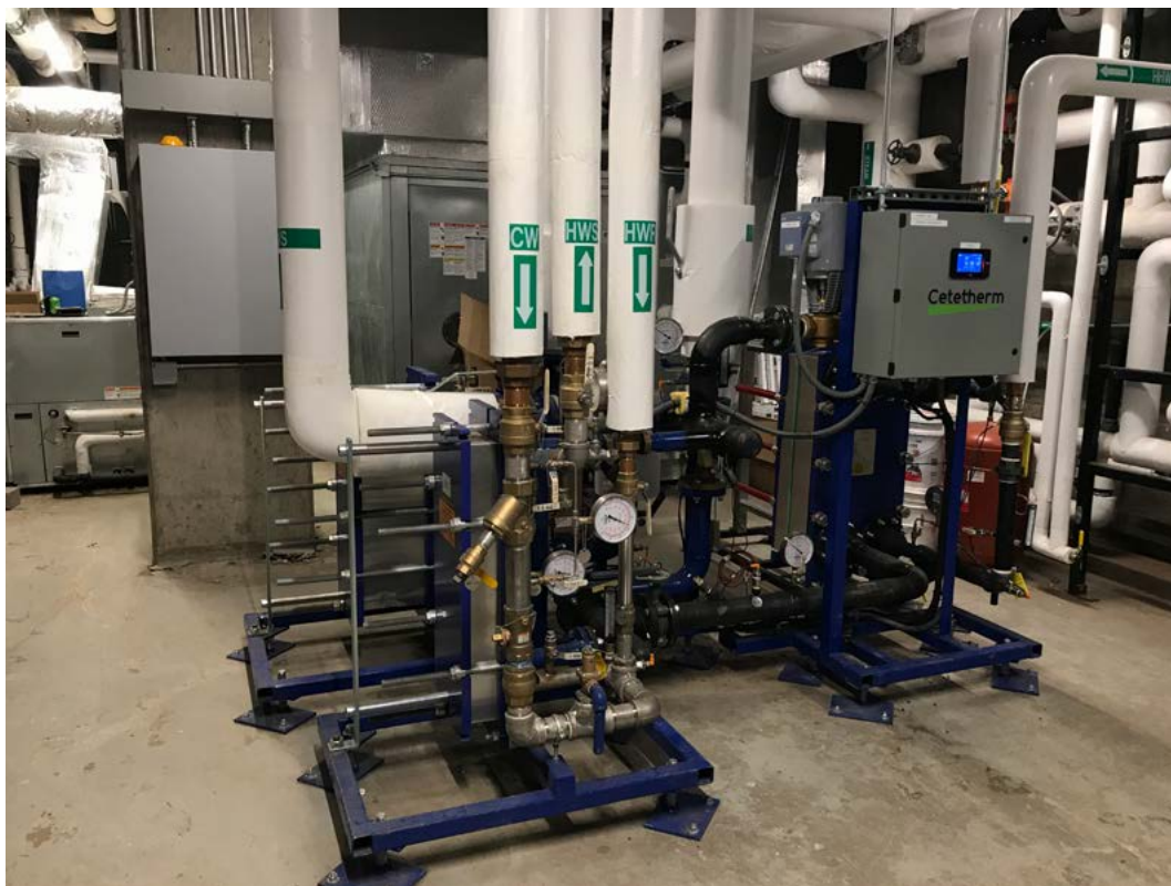
Figure 2. Typical district heating interconnection
